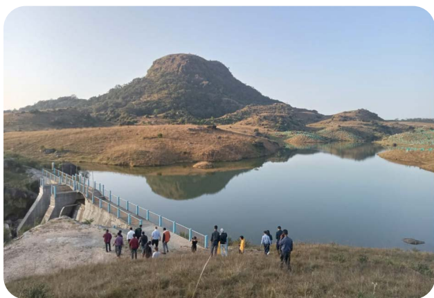
Construction of Check Dam under MGNREGA and Plantation under CLLMP
