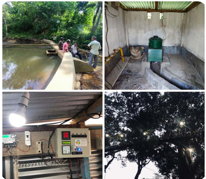
Kudengrim Village in Amlarem Block installed Pico Turbine under Green Energy Mission MINR to light the tourist spot and the streets in the village.
